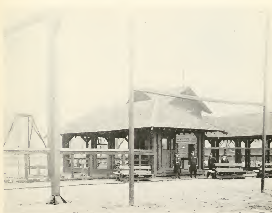
FIELD HOUSE EQUIPMENT AT BEUTNER PLAYGROUND
