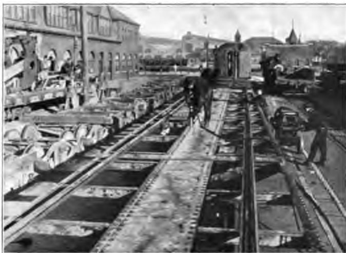
Riveting the underframe
