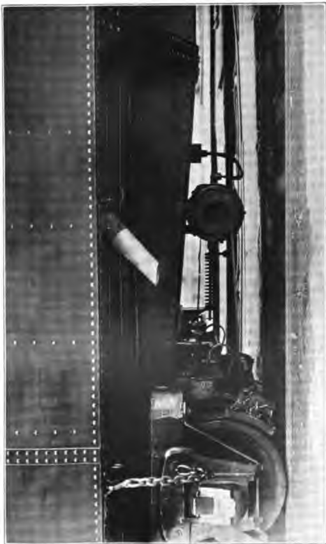
Axle generator for electric lighting of the car
