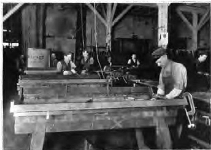
Preparing the steel frame for the upper section of a Pullman sleeping car
